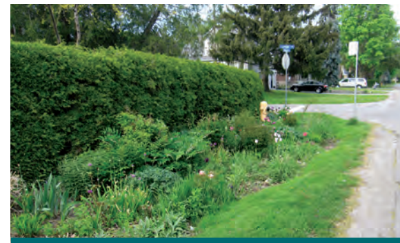
Figure 4.3.4: While many homeowners of this Toronto neighborhood have kept their enhanced swales as grass, a few have turned their swales into gardens that increase stormwater treatment and infiltration. Note that only low growing vegetation was used to avoid encroach on street corner sight lines. (Source: CVC)
