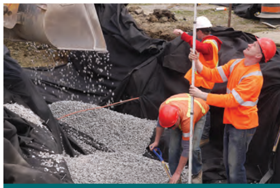
Figure 9.2.2: Contractors verifying the location and elevation of bioretention planters during construction at the Elm Drive Project. (Source: CVC)
