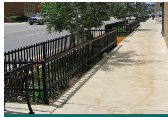
Figure 4.3.32: If grades necessitate a deep bioretention planter, then appropriate fencing should be provided around the planter as was done in this example from Lansing, MI. The Lansing design also incorporated street trees into the planters. (Source: CVC)
