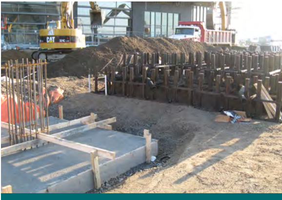
Figure 10.2.3: Proper installation of soil support systems ensures settling does not occur and maintenance is not required. (Source: Deep Root,)
