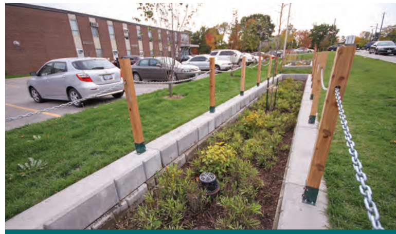
Figure 6.4.11: For bioretention planters with deep, flat-bottomed storage areas, there is more flexibility in placing the overflow spillway because the practice functions as a detention basin, not a conveyance path during infrequent storm events. (Source: CVC)
