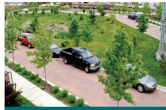
Figure 4.3.16: This light industrial and commercial road in Chicago uses permeable pavers from curb to curb and loops around a dry detention feature. (Source: ICPI)
