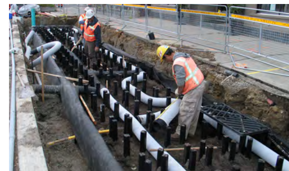
Figure 2.4.3: Installing the soil support system under the sidewalk on part of the Queensway in Toronto. (Source: Deep Root Inc.)
