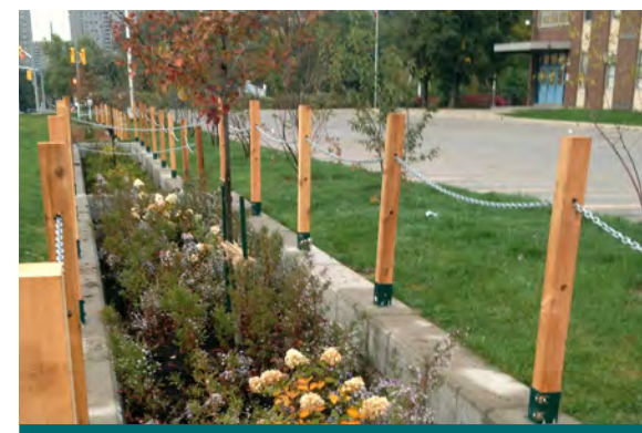
Figure 2.1.2: Bioretention planters aren't just for highly urbanized road ROWs. Planters were used to retain additional road runoff from Elm Drive in Mississauga. (Source: CVC)
