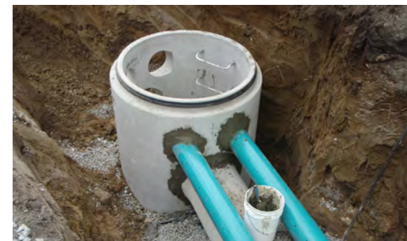
Figure 2.3.1: Perforated pipe systems employ many of the same materials and construction practices as conventional storm sewer pipes, instead using perforated pipes to encourage infiltration during conveyance. (Source: Aquafor Beech)
