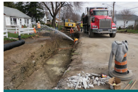
Figure 9.4.2: The costs associated with damage to a pipeline or utility will depend on the type of utility and may include response, repair, environmental impact mitigation measures, and restoration. (Source: Aquafor Beech)
