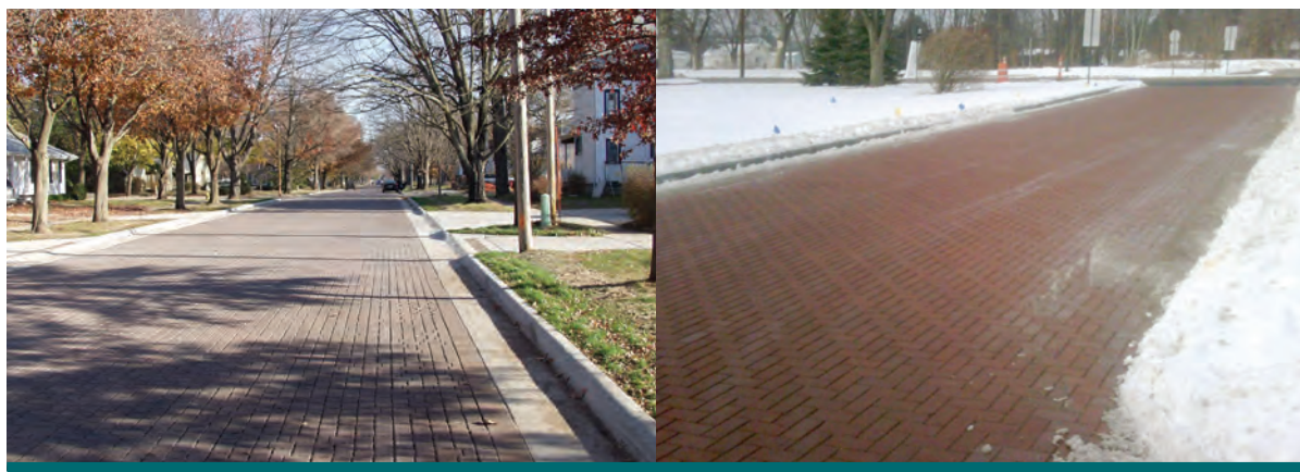
Figure 4.3.7: Permeable pavers used from curb to curb in Charles City, IA (left) and New Albany, OH (right). There are many examples of permeable pavement for the full road within cold climate regions of the US. Snow can be ploughed from permeable pavement as with any other pavement. After ploughing remaining snow can melt immediately into the permeable surface thereby reducing the use of deicers. (Source: ICPI)
