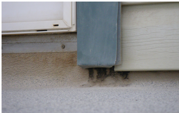
Signs of plasticizer migration from a self-adhered membrane through to the PVC-based liquid-applied membrane.
