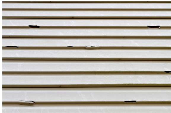
Damage to brittle vinyl cladding during extreme cold
