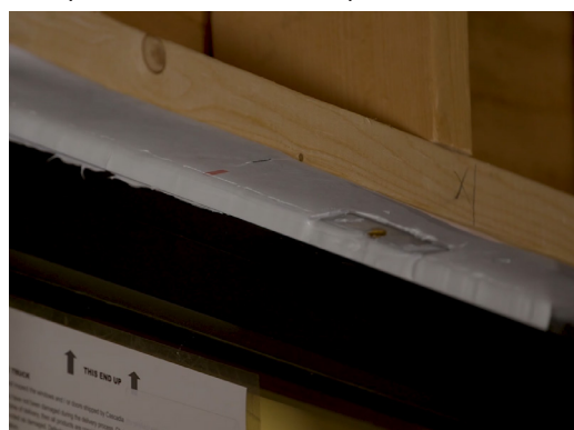
Example of installation with simultaneous tooling of sealant at window perimeter interface.
