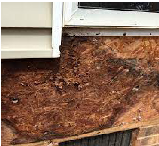
Damaged sheathing due to failure of existing building paper or condensation due to air leakage around windows. Sheathing must be repaired before undergoing a retrofit.
