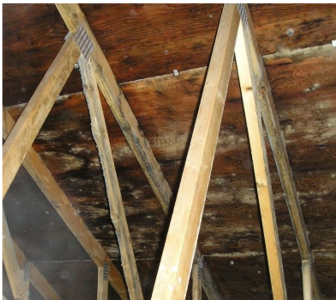
Fungal growth and decay present within attic space requires remediation before undergoing a retrofit. The moisture source must be identified and dealt with and any damaged sheathing and structural framing must be repaired.
