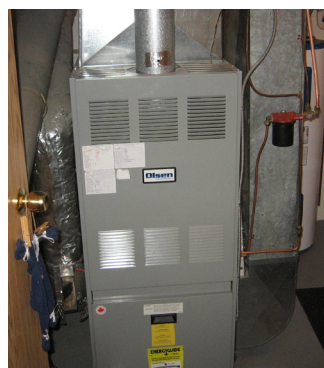
Oil furnace in basement
