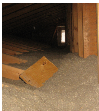
Vented attic with loose fill insulation
