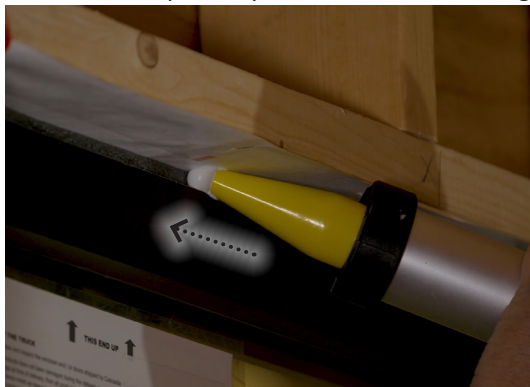
Example of installation with simultaneous tooling of sealant at window perimeter interface.
